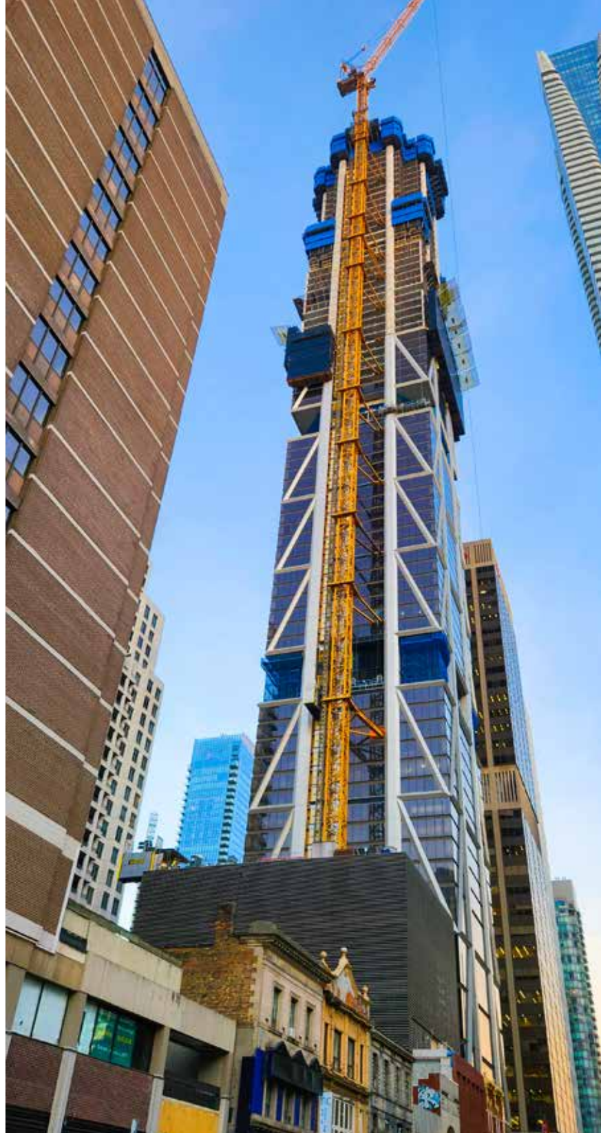
Fig. 1: One Bloor West in Toronto under construction
