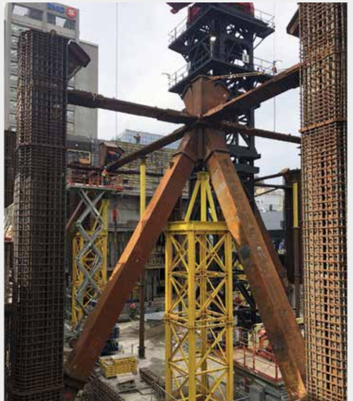
Fig. 4: Erection of mega struts to Level 3 from the ground-floor slab
